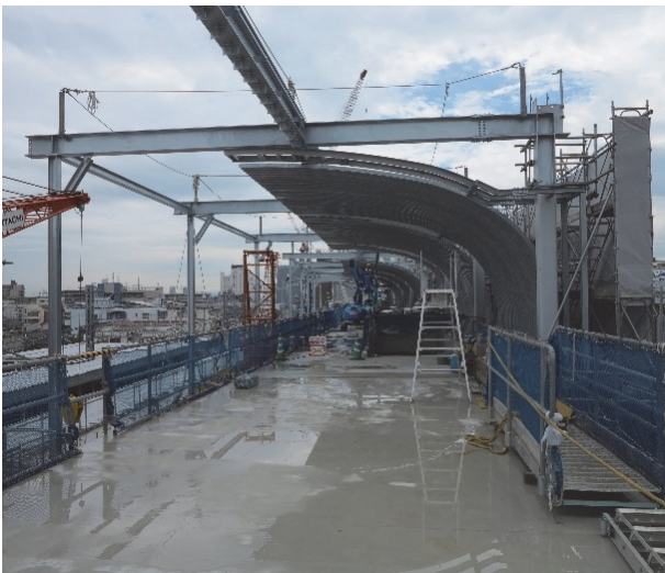
Figure 25. Steel frame before setting up plank sheets
