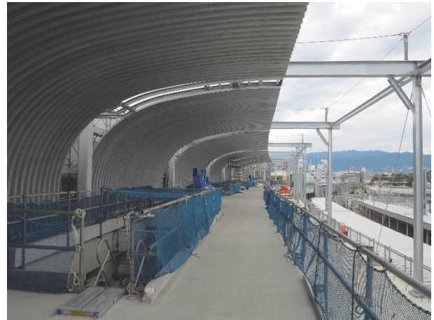
Figure 28. View west of platform
