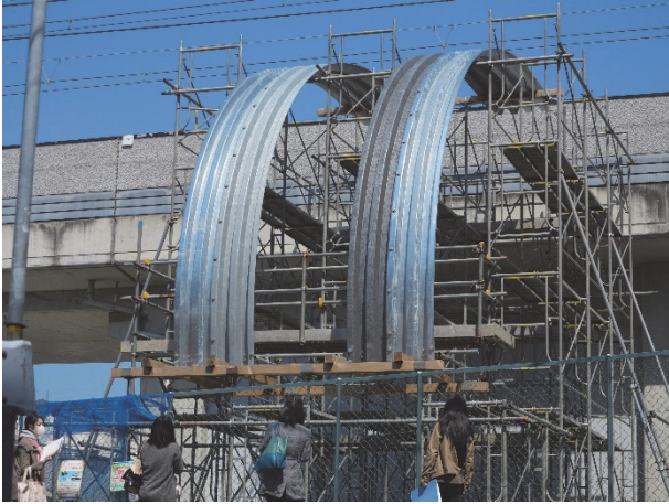
Figure 23. Plank sheet mock-ups
