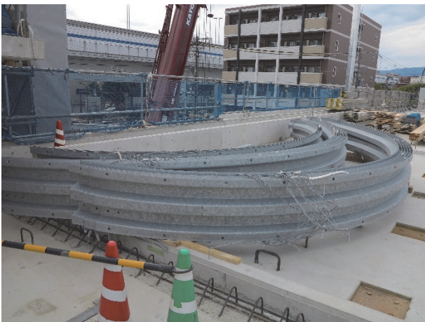
Figure 24. Plank sheets temporarily placed at construction site
